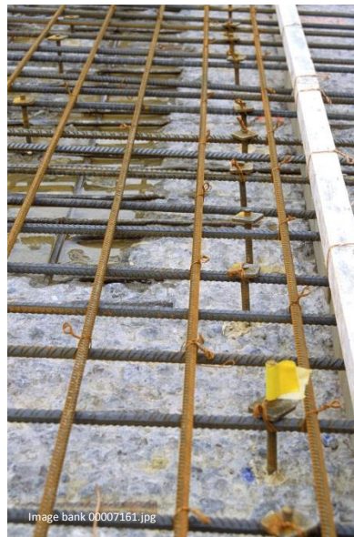
c. Bridge deck augmentation
