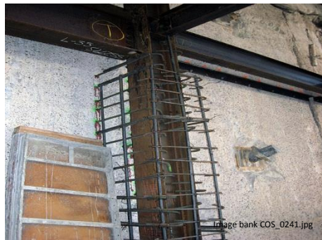
e. Steel column encasement extending from wall
