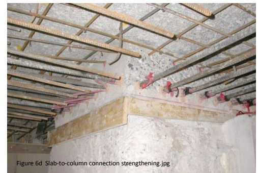
d. Slab-to-column connection strengthening
