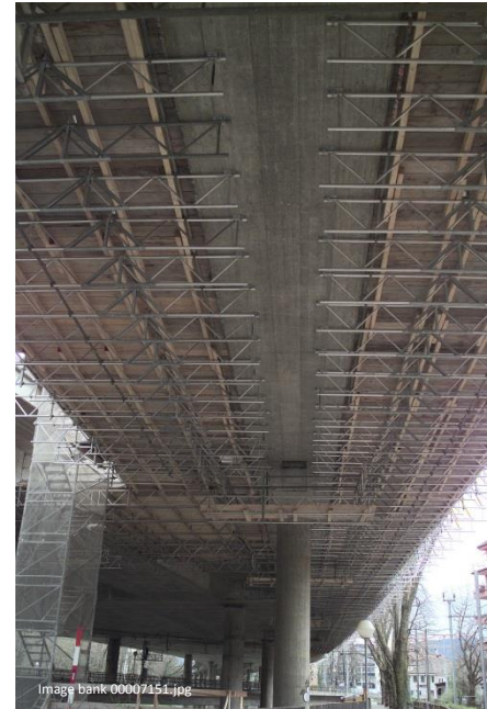
b. Bridge deck rehabilitation
