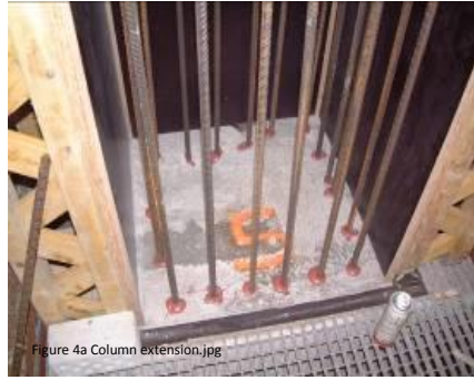
a. Column extension
