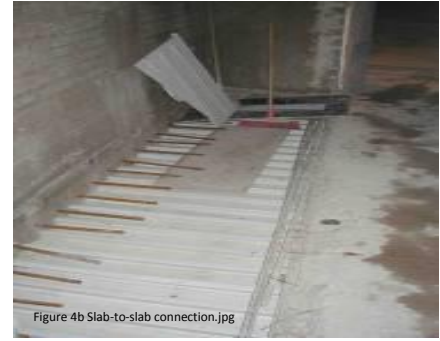
b. Slab-to-slab connection
