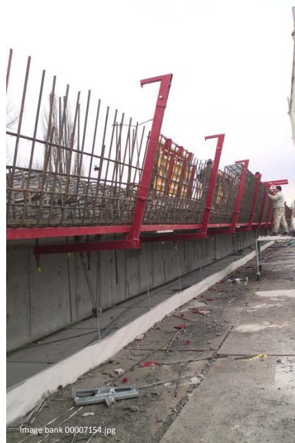
a. Bridge widening
