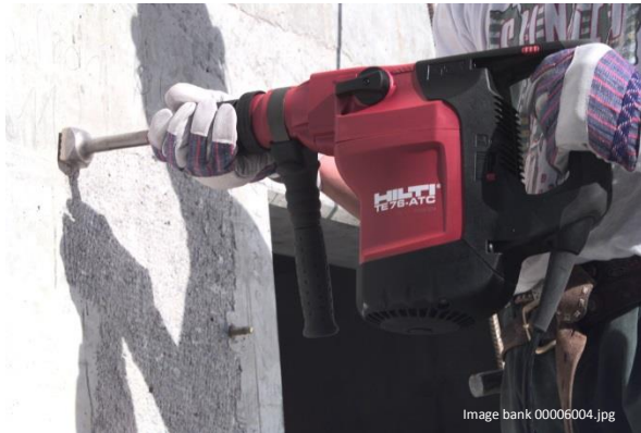
Figure 12 – Roughening a concrete surface with a Hilti TE 76 Combiammer
