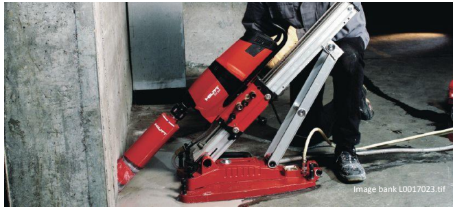
Figure 17 – Inclined core drilling with a Hilti drill stand.
