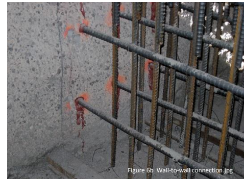
b. Wall-to-wall connection
