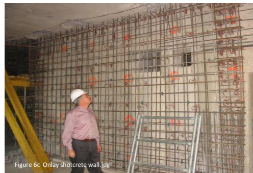
c. Onlay shotcrete wall
