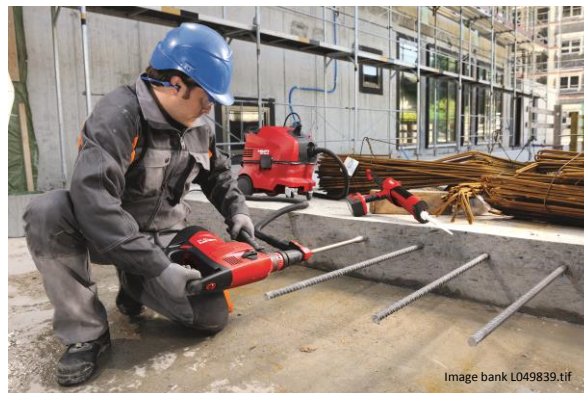
Figure 15 – Drilling with a Hilti rotary-percussive drill equipped with Hilti SafeSet™ technology.
