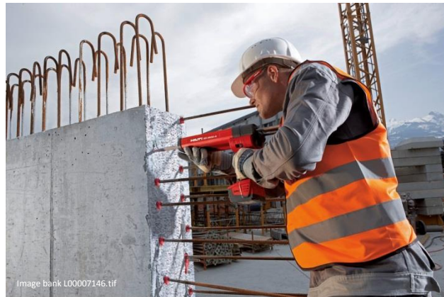
Figure 2– Injecting Hilti HIT adhesive in a drilled hole with Hilti dispenser ED 3500-Ato to simplify installation of post-installed reinforcing bars .
